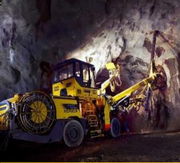
Underground Rock Excavation
