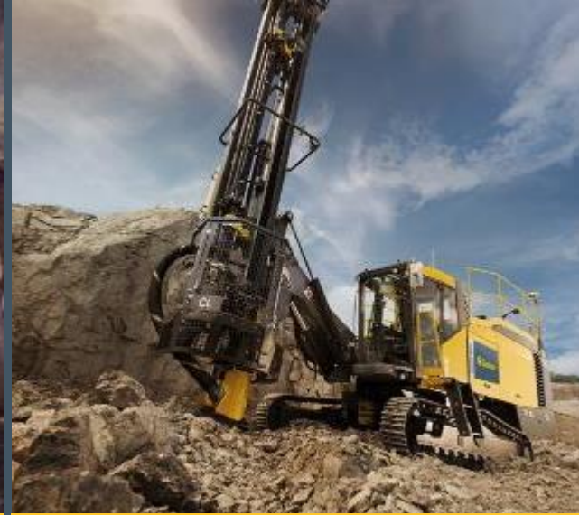
Surface and Exploration Drilling
