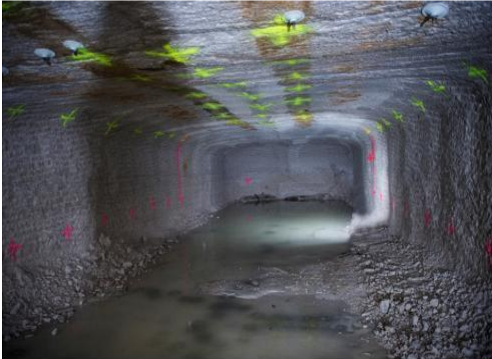
Tunnel by Reef Miner at Atlas Copco test centre, Sweden
