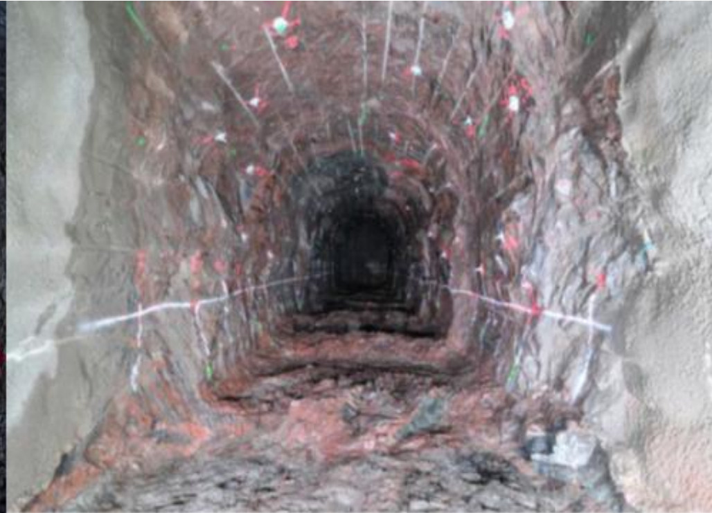
Tunnel by careful blasting at Äspö Hard Rock Laboratory, Sweden
